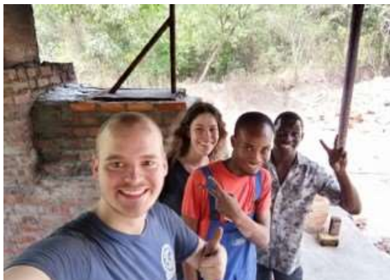
The Project Team in Front of the Repaired Incinerator
