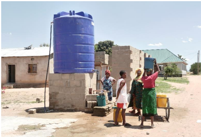
The new well is already attracting many users
