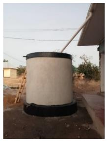
liters and was directly connected to the roof gutter. The water can either be drawn off manually via an outlet at the bottom of the cistern for watering the garden, or by a pipe that was also laid into the building. The cistern has an overflow protection. As part of the project, the pedestal of the drinking water tank from the first project section was also renewed because cracks had formed.
