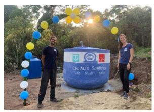
The implemented water supply system collects water from nearby springs in two capture tanks and transports it by gravity through a 2.2km-long pipeline to a cistern with a capacity of 5,000L. The system will provide clean water for 270 people of the Ashaninka tribe, both in the rainy season and in the problematic dry season. The cistern is located at a central and high location
